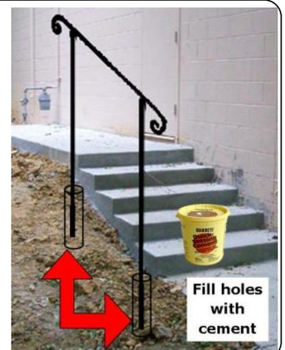
Your EZ Rail comes sprayed with gray primer. This must be covered with rust-protecting paint before or after installation. We recommend painting after installation to avoid nicks. To help your rail stay beautiful for years to come, sand down rust spots and repaint as needed. Contact us with any questions Monday -Friday; 7:00 am - 3:00 pm EST. (412) 221-4488; e-mail: ezrail@verizon.net
